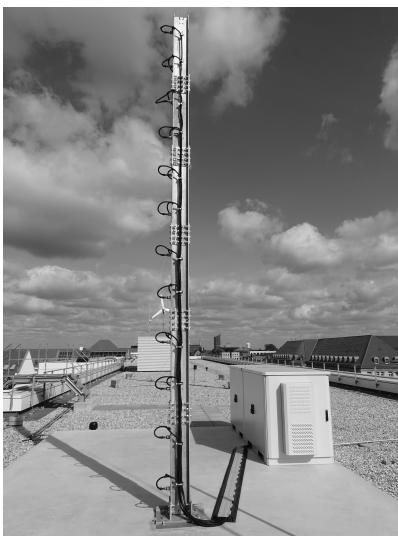
(a) Wind-exposed structure at a rooftop
